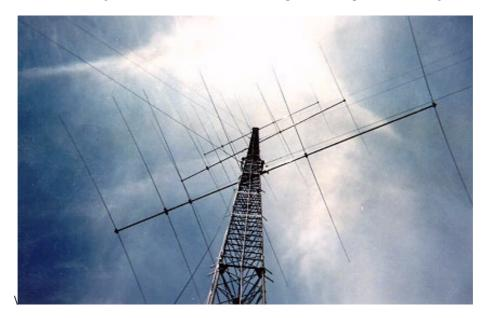
The antenna design was optimized in free space and has the following remarkable characteristics across the band: VSWR < 1.2, F/B > 23dB and Gain > 10dBi.
