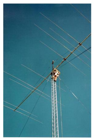
While the 20m performance was unaffected by the interlacing, much optimization had to be performed to bring the 15m statistics back up to their monoband performance. The first major design step was the discovery that the entire 15m antenna had to be placed in front of the 20m driven element in order to get the design to function properly. After this point, computer optimization was used to tweak the antenna to it final stage.
