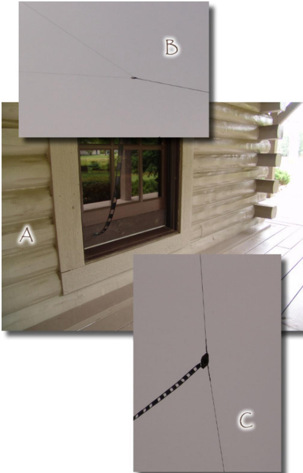
**A** - Method used to bring 450 ohm feed line into the shack consisting of a painted 1 x 6 board cut to the window's width. The feed line passes through a slot. Clear silicon sealant was used throughout.
