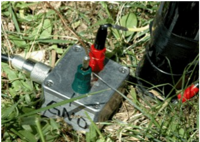
Coax to System Hookup Box
